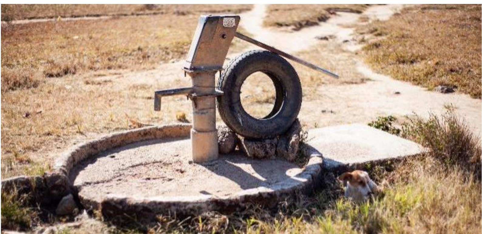
Figure 10: An abandoned borehole at LEA Primary School Tabore. Photo credits CRADI 2024
